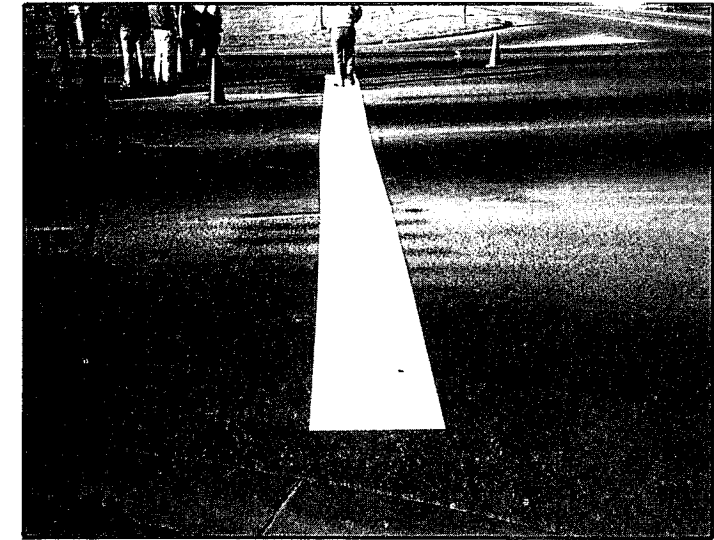
3M coldplastic material being installed
